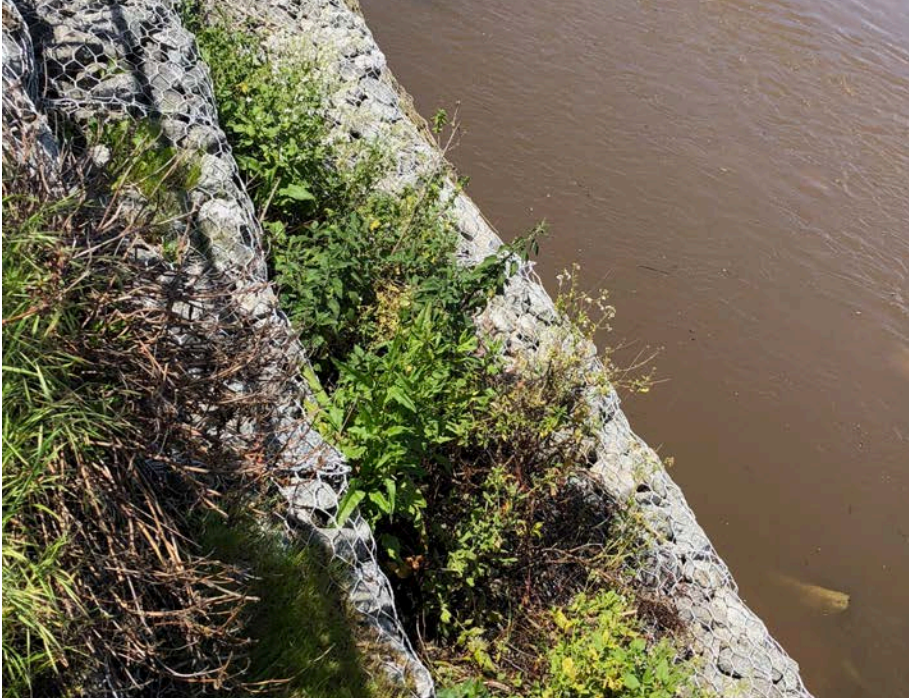
Stone riprap levees line the riverbanks.
