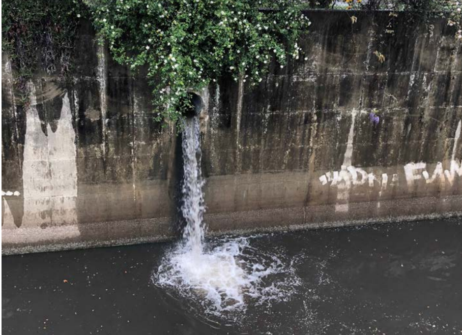
After a rain, storm-water runoff empties directly into the river.
